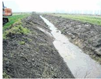
During ... Re-battering of the drain.
