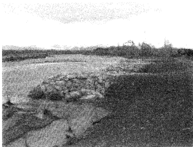
Figure 45.2 Stub rock groynes and pole planting upstream of a highway bridge, Hurunui River, North Canterbury.
