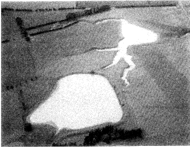
Figure 19.7 Off-stream storage reservoir in the Glenmark Irrigation Scheme near Waipara, Canterbury. The water is held in the nearer reservoir by a constructed embankment about 4 m high on three sides; the further reservoir is held by a barrage across a topographic depression, but both are fed by inter-basin transfer from Weka Stream. Other reservoirs in this scheme are contained entirely by embankments. Photo: Paul Mosley
