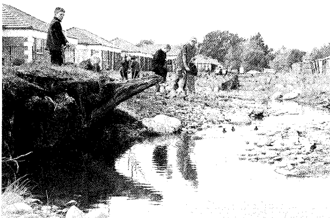
Figure 38.9 Large hardwood tree stumps were placed upside-down in the banks of Papanui Stream in Christchurch to create a stable overhang and interesting landscape feature.
