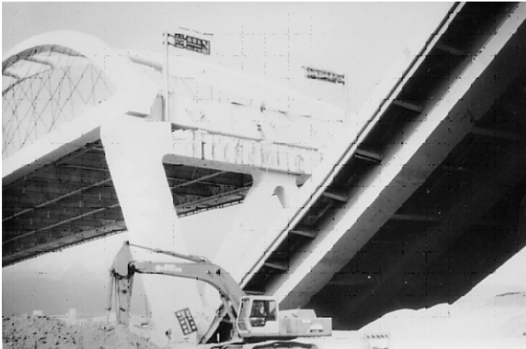
Fig. 14 Loss of Approach Span of the Nishinomiya-ko Bridge (Kobe, 1995)
