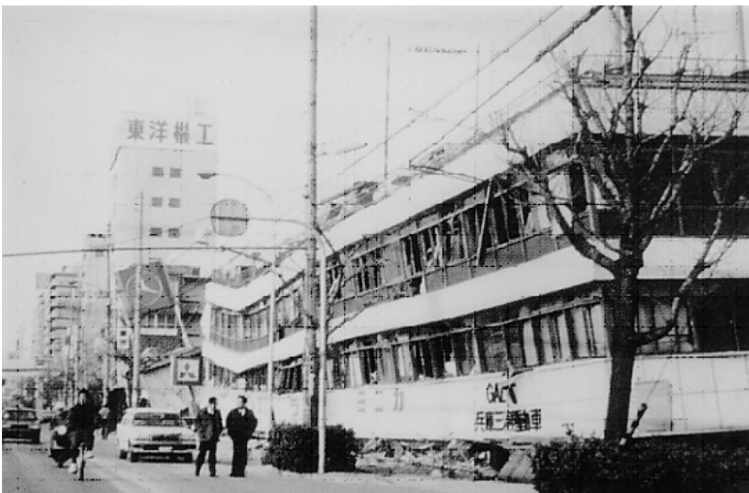
Fig. 9 Soft Storey Collapse of the First Storey of a Departmental Store (Kobe, 1995)
