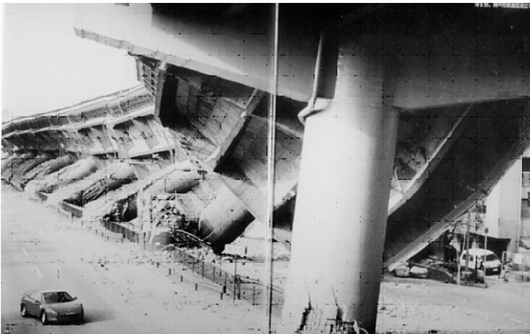
Fig. 15 Failure of Columns of the Hanshin Expressway Near Ashiya (Kobe, 1995)
