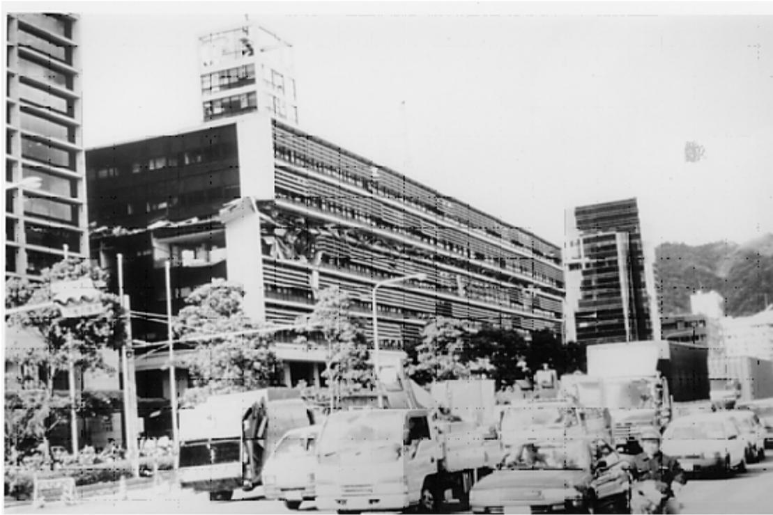
Fig. 10 Soft Storey Collapse of an Intermediate Storey of a Municipal Building, (Kobe, 1995)
