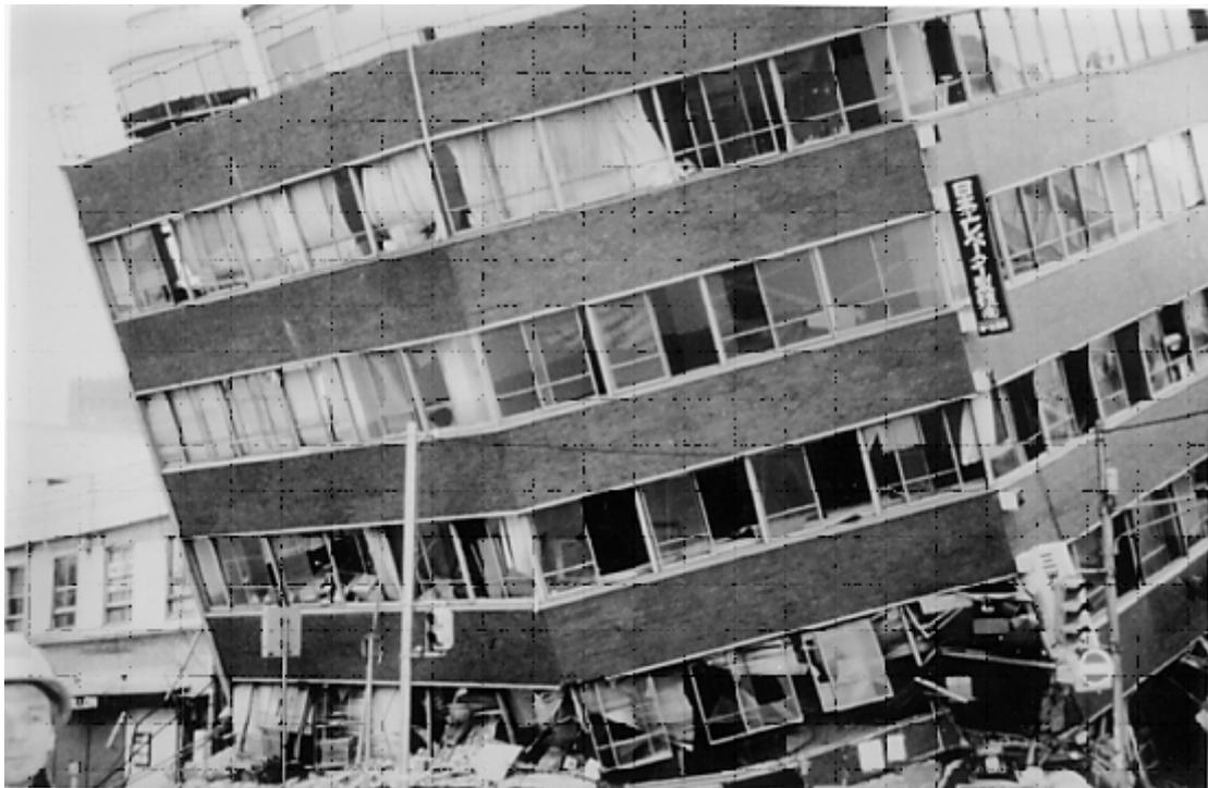
Fig. 11 Collapse of a Building With an Unsymmetrical Structural Configuration (Kobe, 1995)
