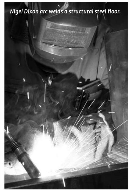
*Nigel Dixon arc welds a structural steel floor.*
