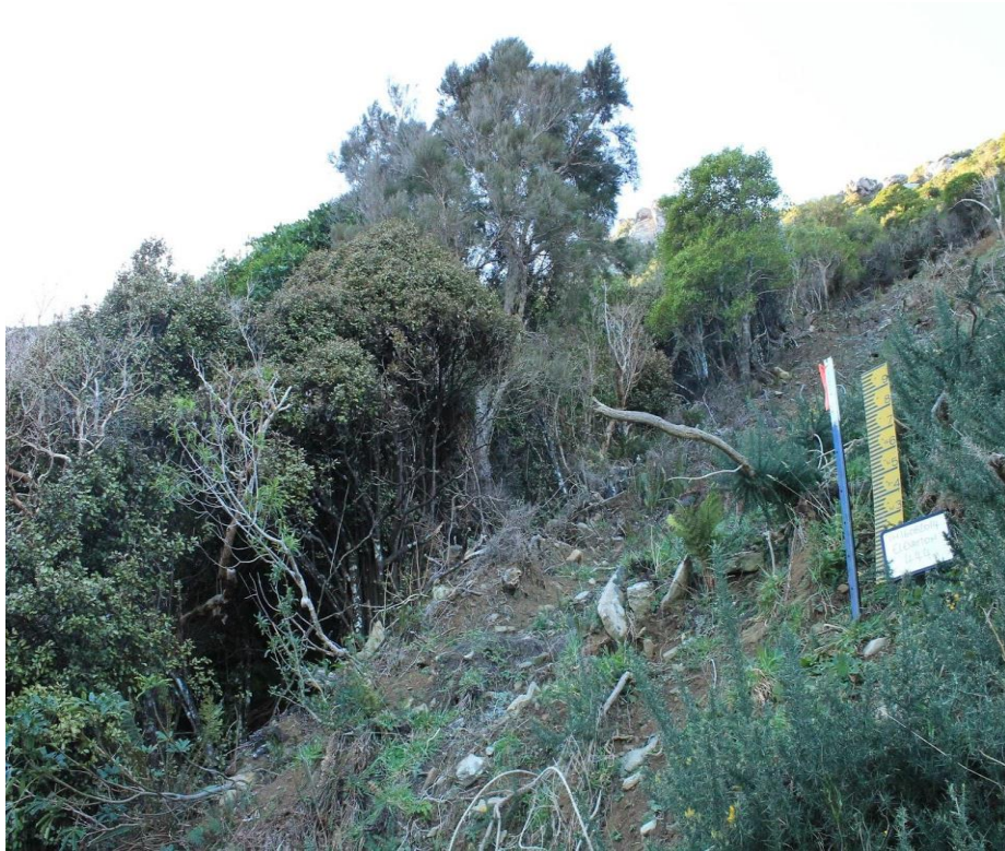
Figure 8. Landslip above lodge on face of Panama Rock.
