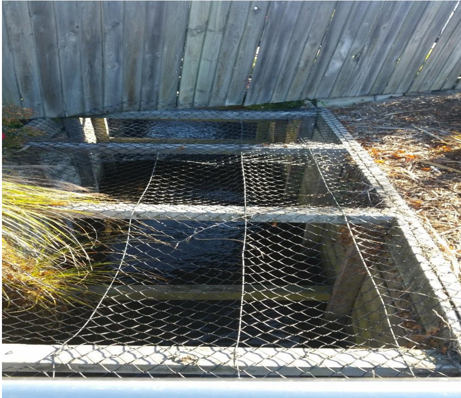
Figure 10: Board drain in Riccarton, Christchurch.
