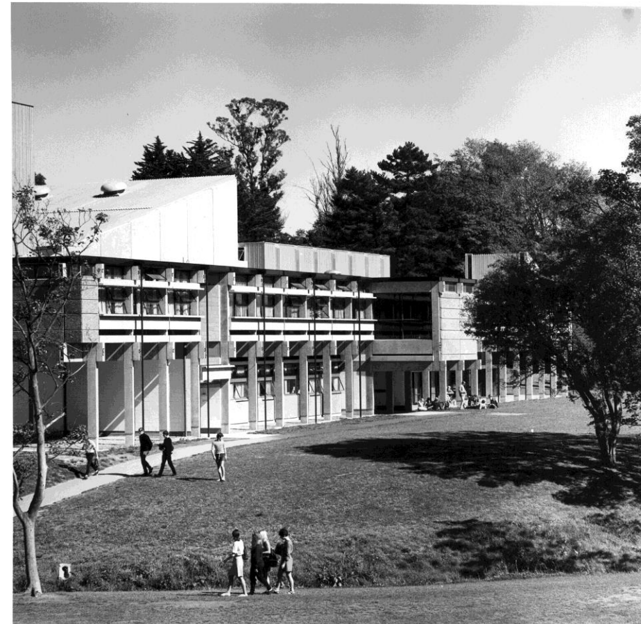
UCSA Building: date unknown
